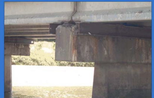
2000 Repair To Support Bridge Deck
