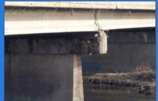
Concrete Spalding of Bridge Deck Support
