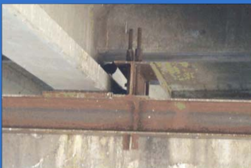
2000 Repair To Support Bridge Deck
