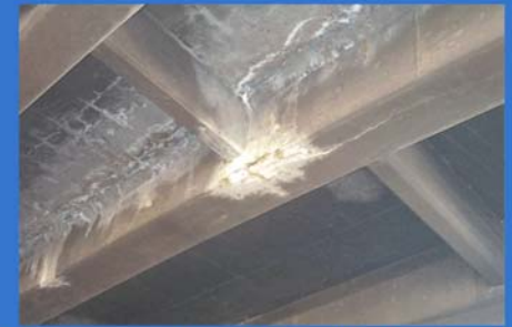
Concrete Spalding of Bridge Deck
