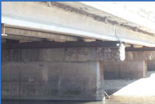
Concrete Spalding of Bridge Deck Support
