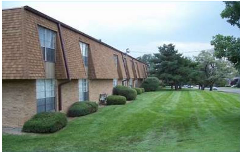
Aztec Village Apartments offers affordable rental units.
