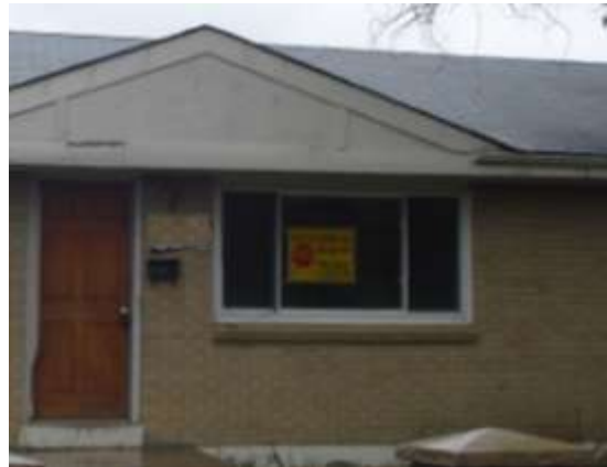
A foreclosed/vacant HUD home in Thornton
