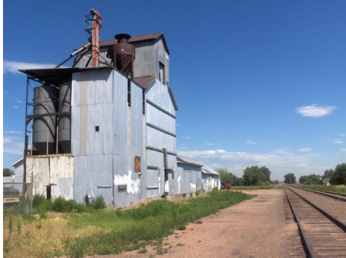
The Eastlake grain elevator is being evaluated for nomination as a historic landmark.
