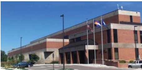
▲ Wes Brown Water Treatment Plant
